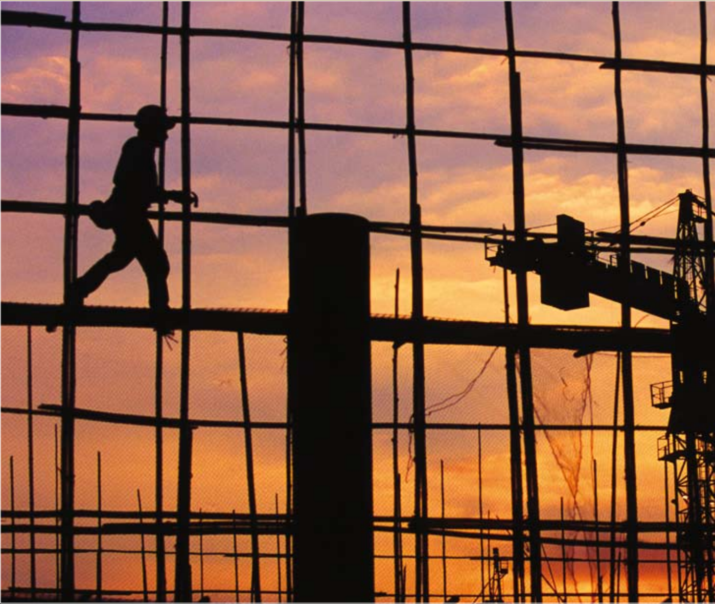
Balancing deftly on high-rise bamboo scaffolding in HONG KONG SAR
